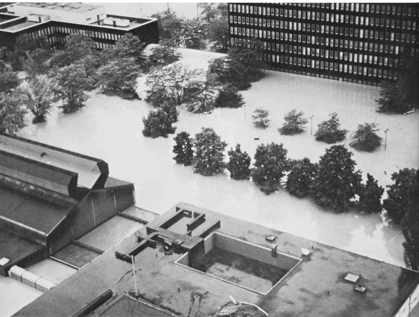
Aerial view of the Corning Museum of Glass surrounded by flood water, June 23, 1972.
